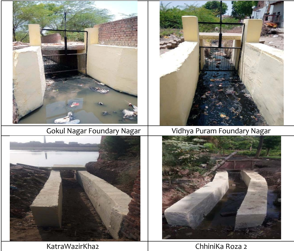
FigureA1.50: Drain Barrier in Agra
