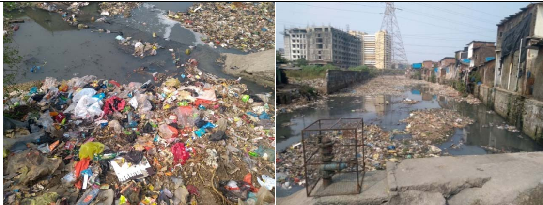
Drain Near Mankhurd Station (19°02'54.7"N 72°55'57.1"E)-Picture depicting plastic Clogged into Drain
