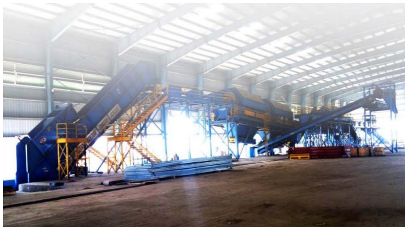
Photo Plate No.4.26 Material Recovery Facility (MRF) at Kanjur Processing Plant.
