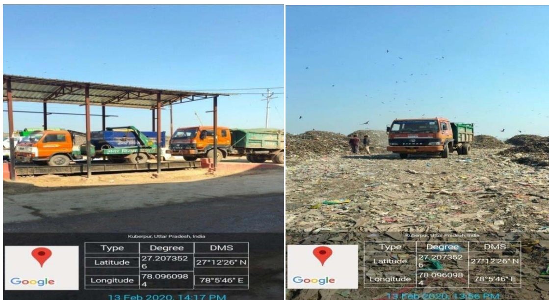
Figure A1.19-Transfer of Waste from Transfer Point to Disposal Site
